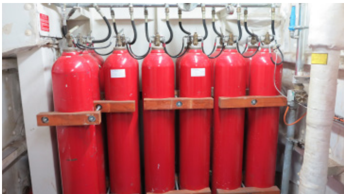
Increased capacity of the CO 2 system is necessary for methanol (has bound oxygen).
