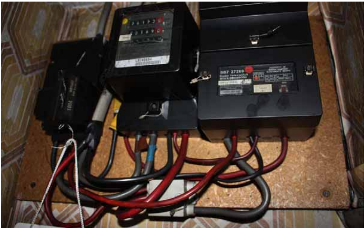
Image showing that cut out fuse and meter were not involved.
