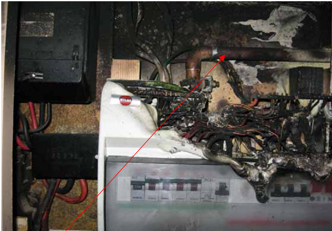
22mm gas pipe running immediately behind distribution board.
