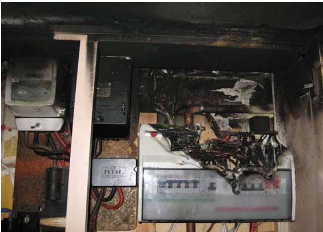
22mm gas pipe running immediately behind distribution board.
